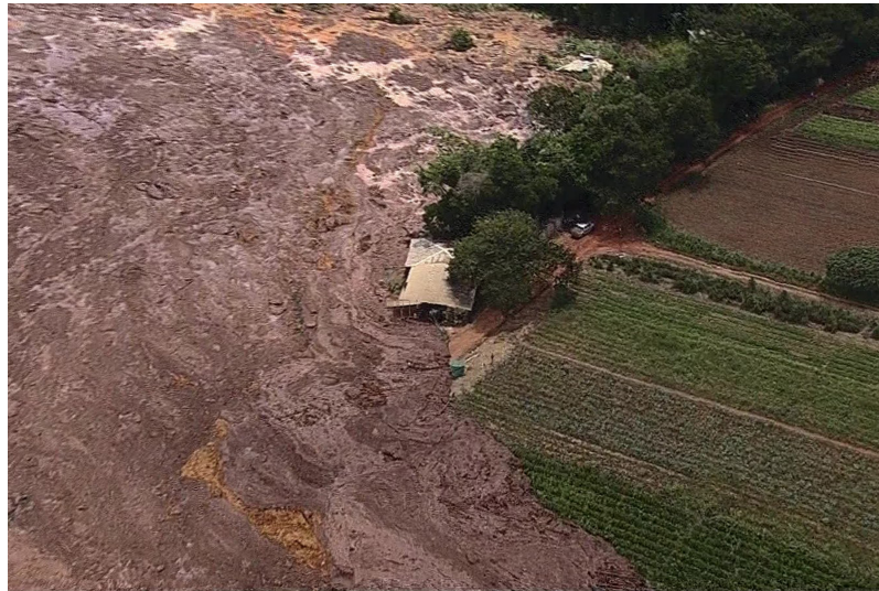
Fig. 1. Deadly mining dam collapse in Jan 2019 at Brumadinho, MG. Brazil [Times 2019]
